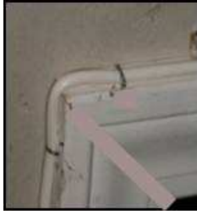
Figure 3 - Picture of EZ Bend stapled around a doorframe
